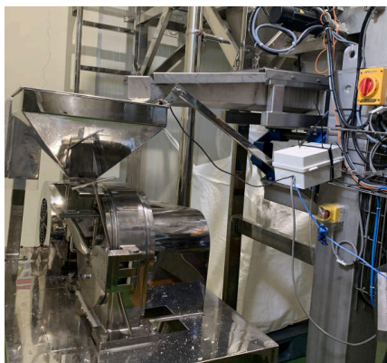
Feeding unit of a drying line, before commissioning.
