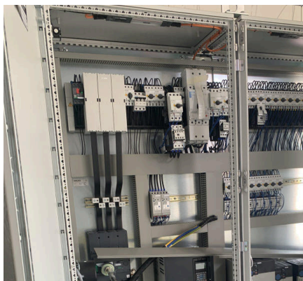
Wiring the control panel during installation.
